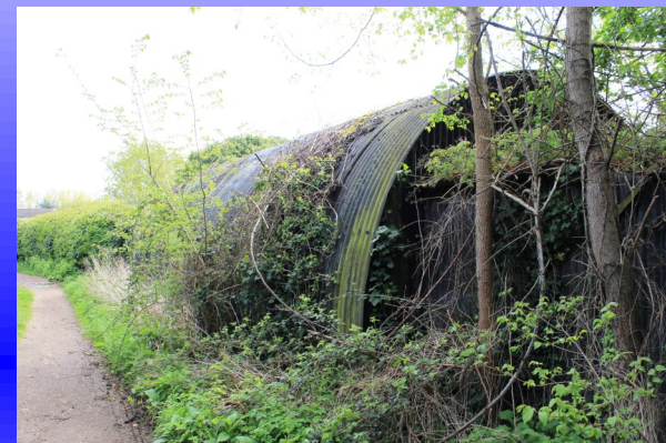
Old Nissen Hut on path from Orchard to Lode Way
